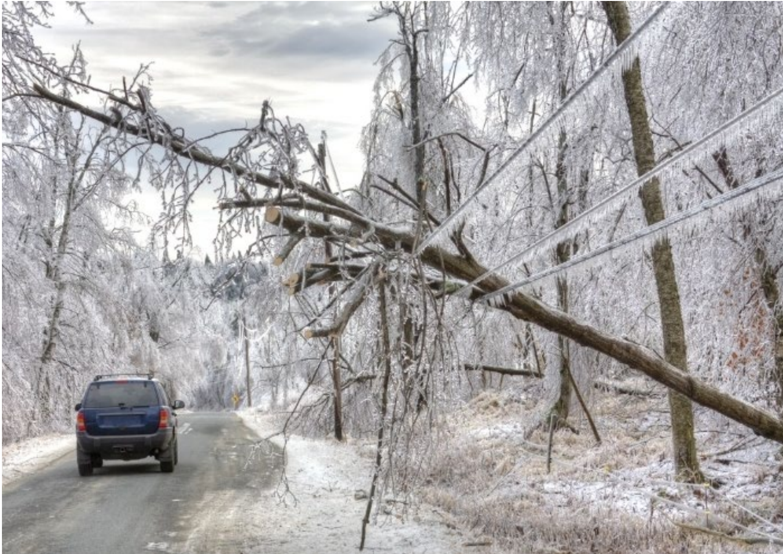
Ice storm impacts power lines
